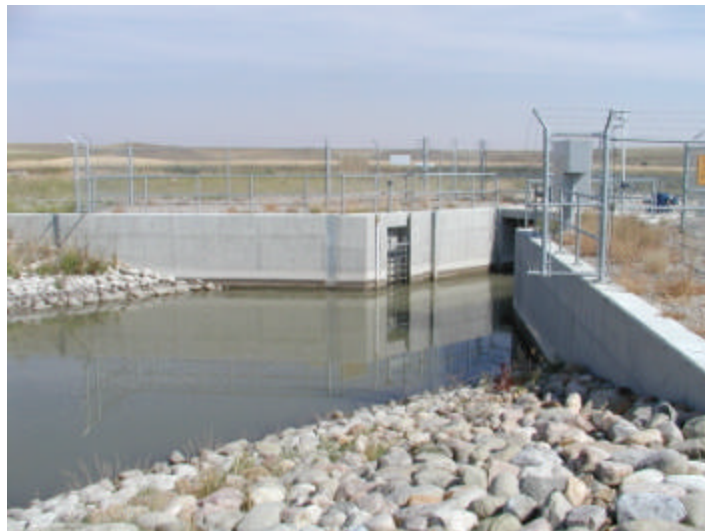
Diversion Structure on Mosquito Creek (photo taken 2003)
